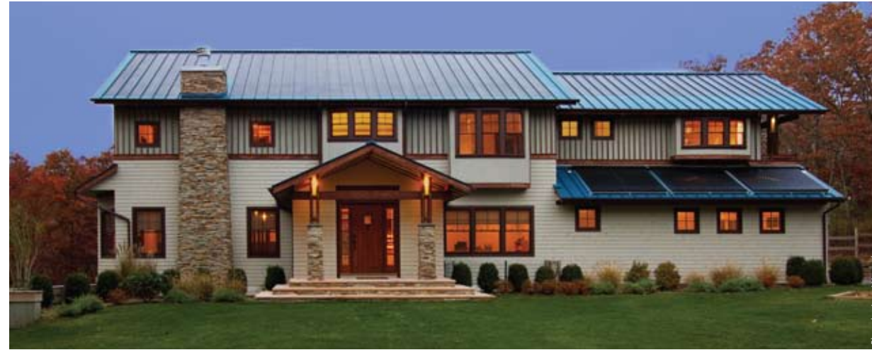
Telemark's HGA House (Hamptons Green Alliance) is a USGBC-LEED Platinum home and received special recognition from the NYS Senate and NYS Assembly.
